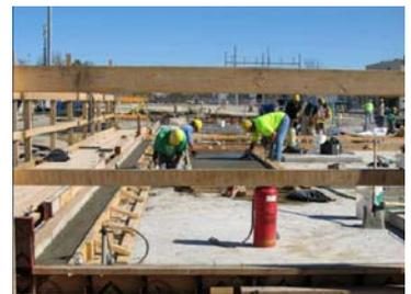
Equipment pads being placed for SCWO Processing Building
