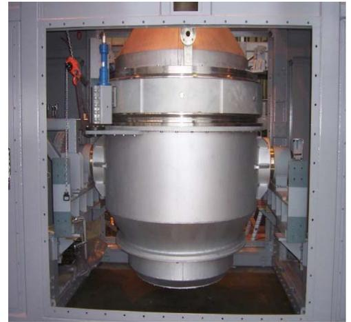
The Static Detonation Chamber
